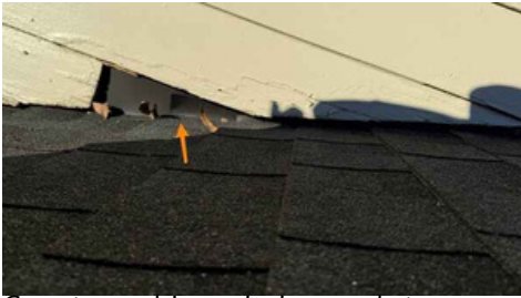
Counter flashing missing, and step flashing is bent out and exposed
