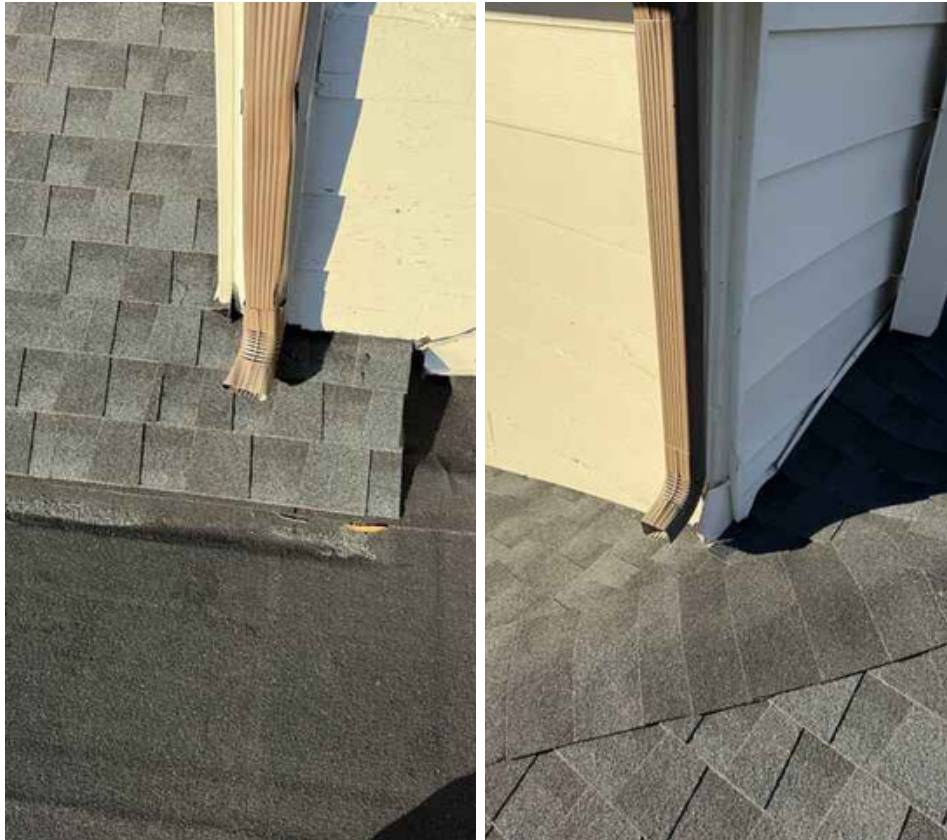
Gutter Improperly Discharging onto Roof
