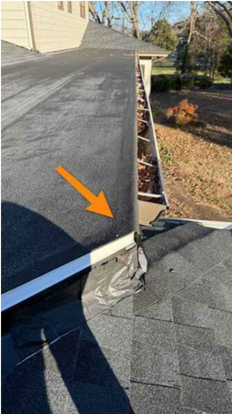
Flashing and corner needs to be repaired.
