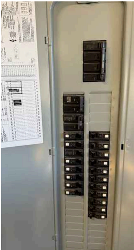
Main & Subpanels, Service & Grounding, Main Overcurrent Device: Panel Capacity 200 AMP
