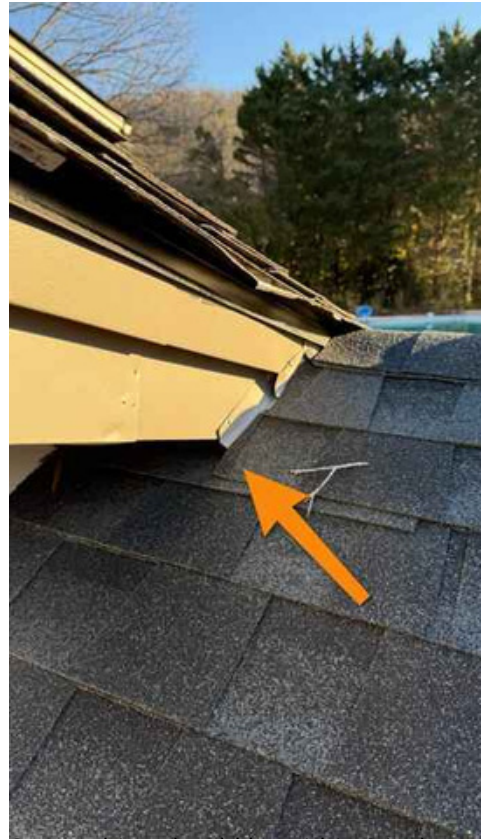
Step flashing should be within 2 inches of the end of the shingle.
